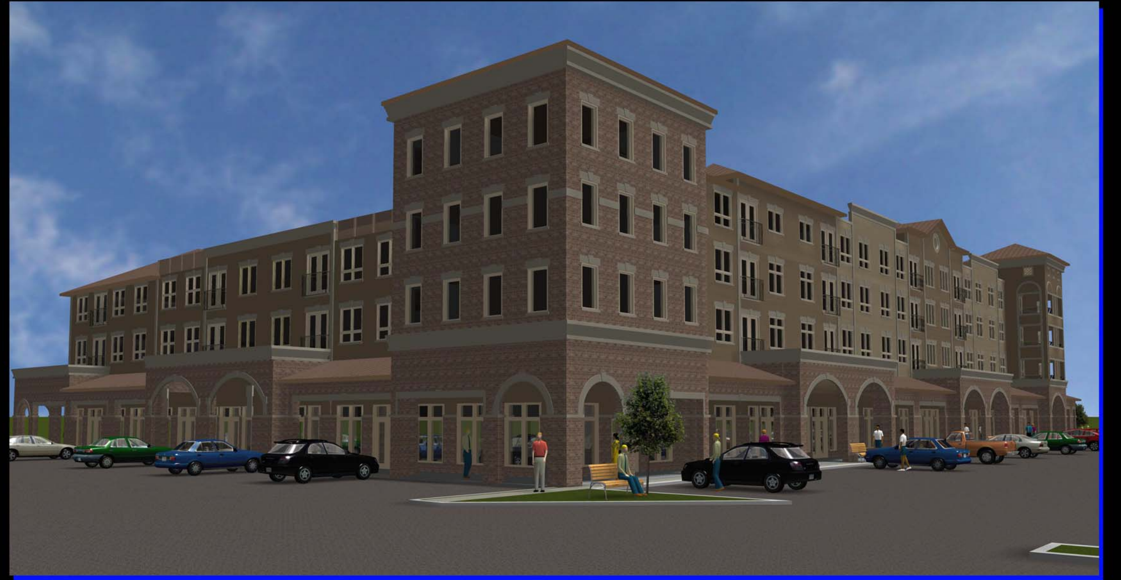
North - West Corner (Princess Street & Centennial Street)
